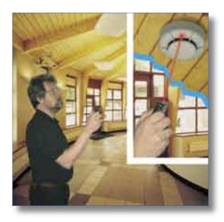
Routine testing has traditionally involved physical access to the installed unit, a time-consuming procedure often requiring the use of step ladders or long poles. The ECO1000 is tested from ground level using a laser based remote alarm test unit. The commissioning or service engineer directs the modulated laser beam at the detector's LED; the unit responds to the commands and latches into alarm. What could be simpler?
